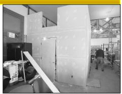
having priority, was completed first. The drywall was taped, mudded and painted. The floor was tiled, molding applied and fixtures installed. Lights and fan were installed as the janitor room was finished. Doors were put on and the exterior walls were paint-
