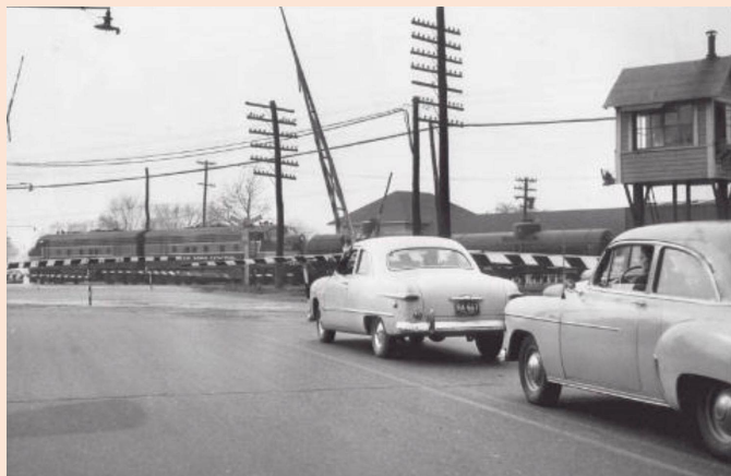
Vine Street RR crossing before underpass
